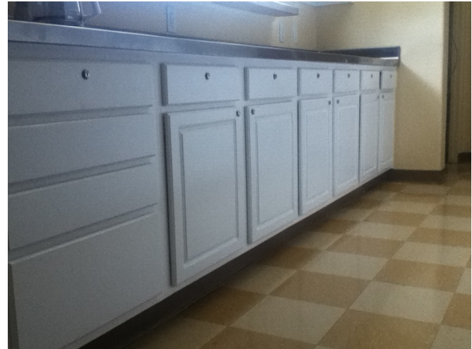
Re-finishing cabinets and painting kitchen
